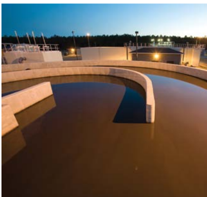
If capital investment and O&M spending for wastewater infrastructure remain at current levels, EPA estimates a funding gap of approximately $270 billion 2000–2019. (Photo by Jerry Blow Architectural Photography)
