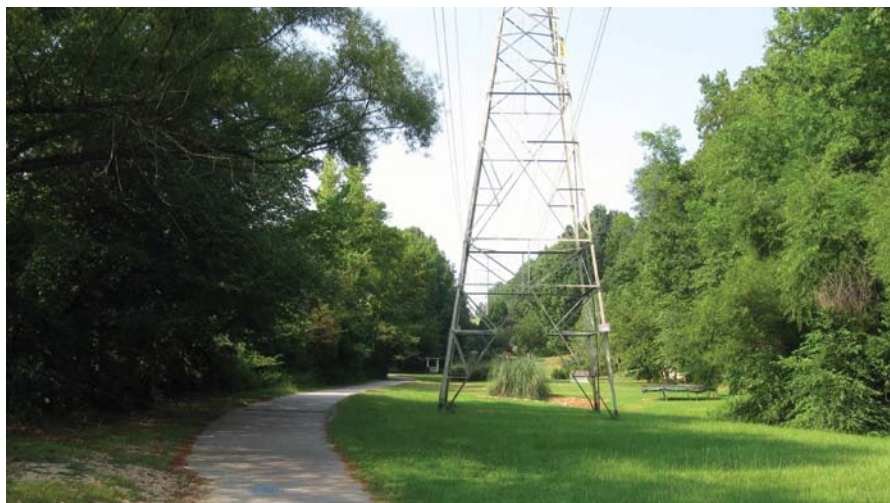
Above-ground electric transmission lines and buried large-diameter water and sewer mains make accurate above- and below-ground location essential.
