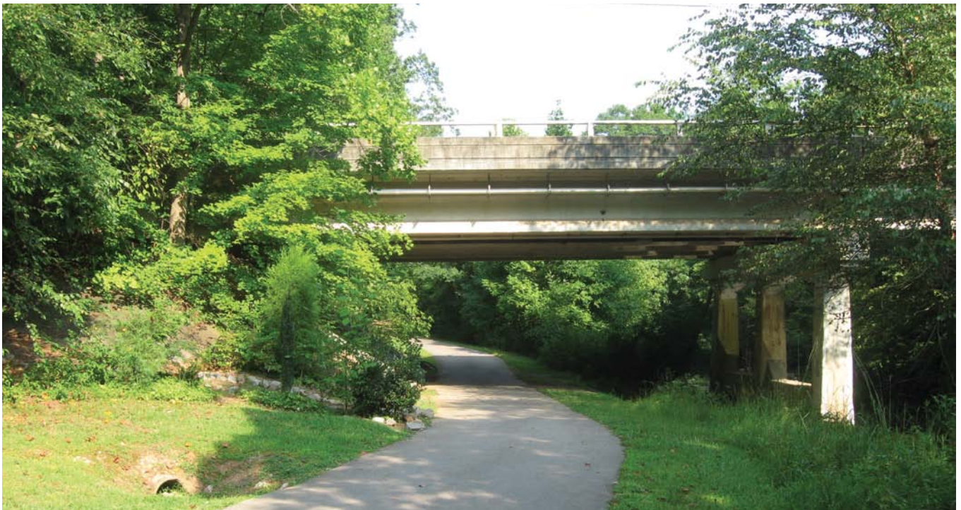
Tunneling will be required to install the gravity sewer under some of the roadway bridges along the alignment.
