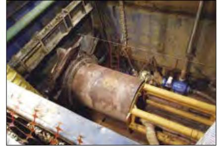
*Shown here is the microtunnel boring machine and casing pipe contained in the tunnel's launching shaft near the outfall crossing at US Highway 501. This marked another first for the City of Durham and the NCDOT's Durham District.*
