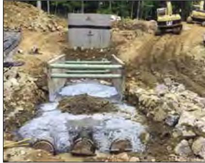
*This is one of the three Eno River crossings shown halfway complete with recently poured concrete encasement.*
