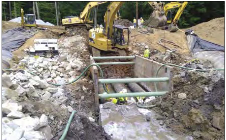
*This is one of three Eno River crossings. It included cofferdam installation, riverbed removal, and installation of three 24-inch diameter ductile iron pipes which are the hydraulic equivalent of a single 48-inch outfall.*
