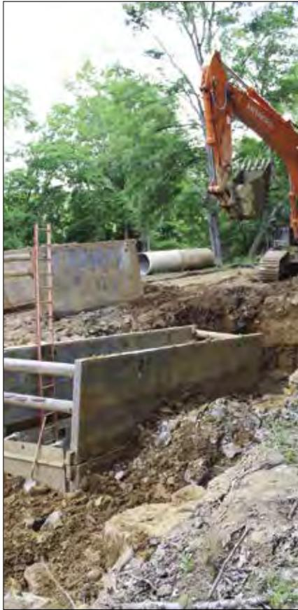
Trenching for the new outfall pipe involved the use of an excavator that was shipped to the site and assembled prior to mobilization. Trenching also included drilling and blasting of rock for removal, and installation depths in some places of up to 28 feet below grade.
